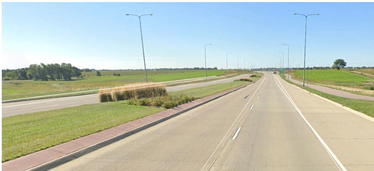
Figure 7. Street view of North Veterans Parkway offers example of what South Veterans Parkway would look like from the road.
