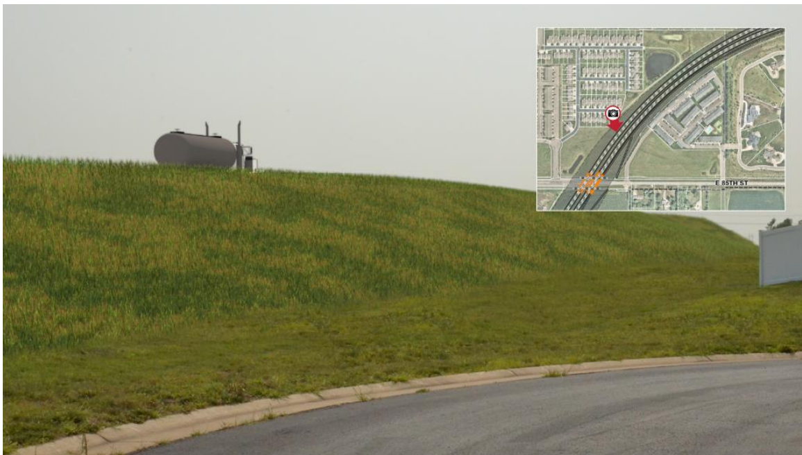
Photo 6. The southern viewshed distance from Harmody Estates would be reduced by the road fill required to construct the 85 th Street overpass. The embankment consists of prairie grasses. 85 th Street and power lines would no longer be visible off in the distance. Traffic would be noticeable, particularly in the outer lane nearest to the cul-de-sac. Much of the traffic within the inner westbound lanes and eastbound lanes would be shielded as a result of the embankment.
